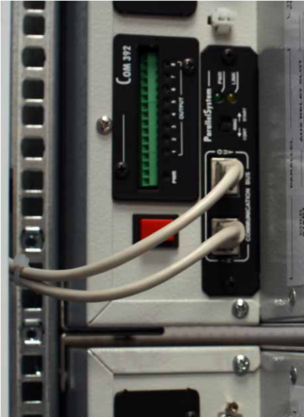
Parallel configuration and programmable relay contacts board
